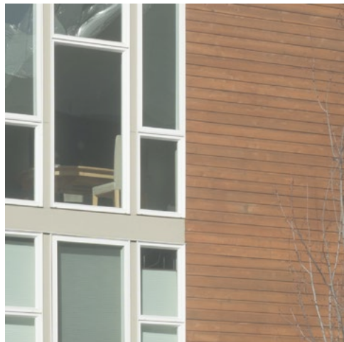
DC-4: Wood siding/vinyl window with FCP spandrel
