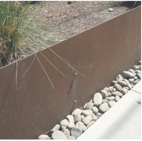
DC-2: Retaining wall at sidewalk
