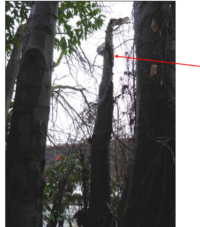
Photo 1: Red alder tree 190 looking east. Arrow points to large column of decay in trunk leaning over Westlake Ave N.
