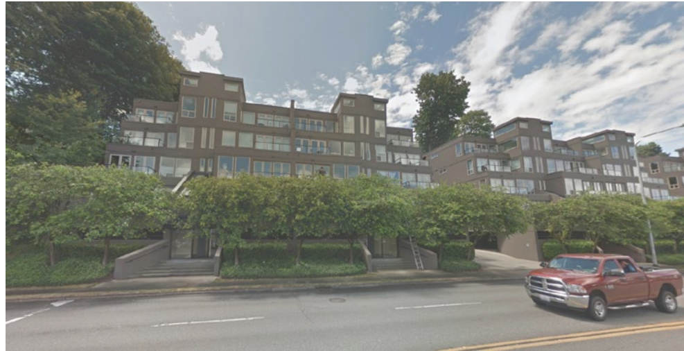
D 2105 Westlake Ave N - Multi-Family Residence
