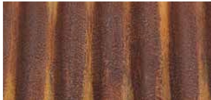
^ corrugated, preweathered steel siding
