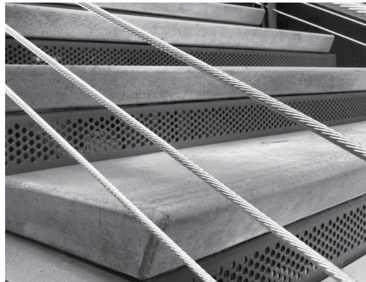
^ precast treads and steel risers
