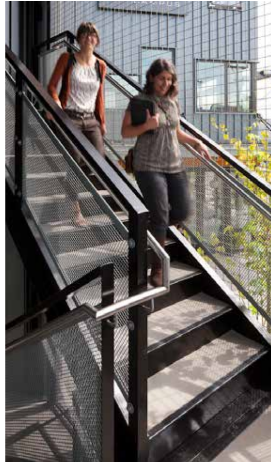
^ open mesh wall & black steel rail
