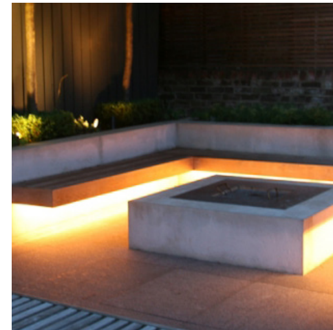
RECESSED STRIP LIGHTING
