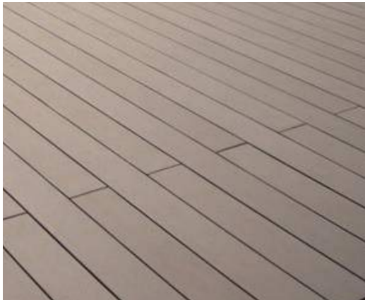
Option 2- 12" wide pultruded plank paving (in ROW, Option 1 to be used)
