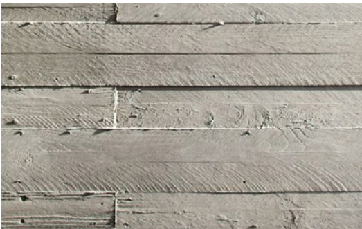
Concrete Boardform Site Walls
