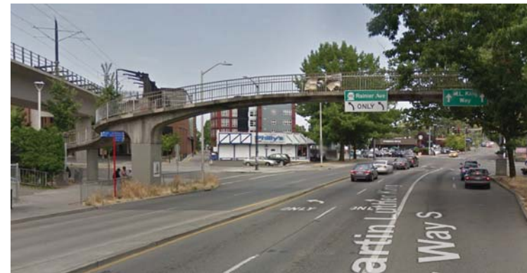
7 Elevated pedestrian bridge
