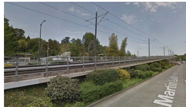
8 Elevated train track
