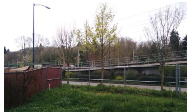
5 Elevated train track
