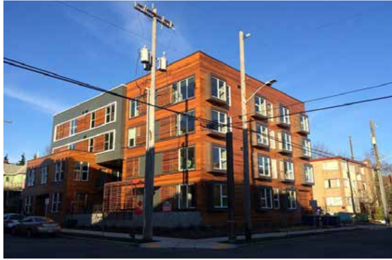
③ Yardhouse Apartments Built: 2014, 35 units
