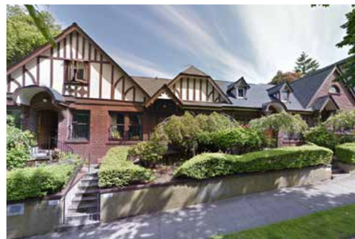
7 1300 E. Mercer St. Apartments Built: 1926, 8 Units
