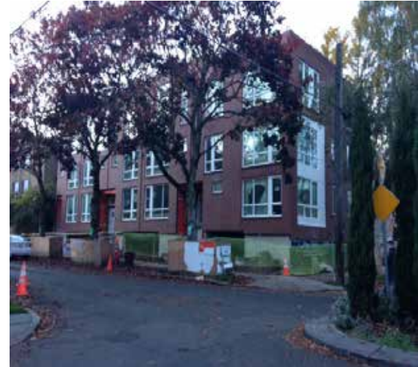
④ Mercer Rowhouses Built: 2015, 5 units
