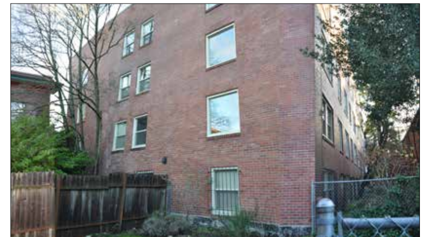
⑦ View West of the Fairhome Apartments building
