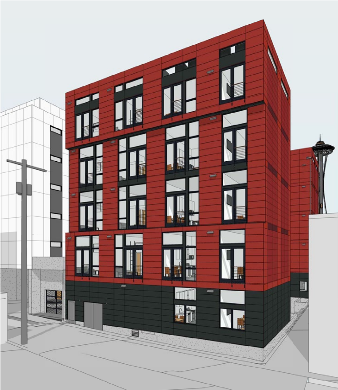
Building perspective from the alley looking northeast: The building is stepped back at levels 3 and 4 to provide powerline clearance as required by Seattle City Light.
