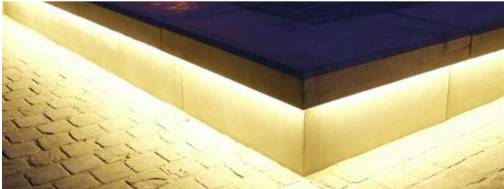
CONCRETE PLINTH BENCH SEATING (C.I.P.) WITH LED LIGHTING AT REVEAL
