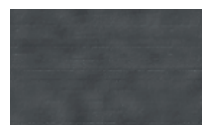
textured boardformed concrete
