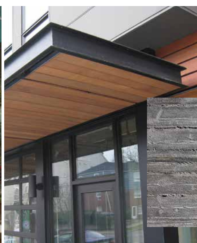
^ entry canopies with steel frame and cedar soffit
