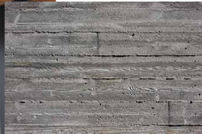
cast-in-place concrete with boardformed texture v
