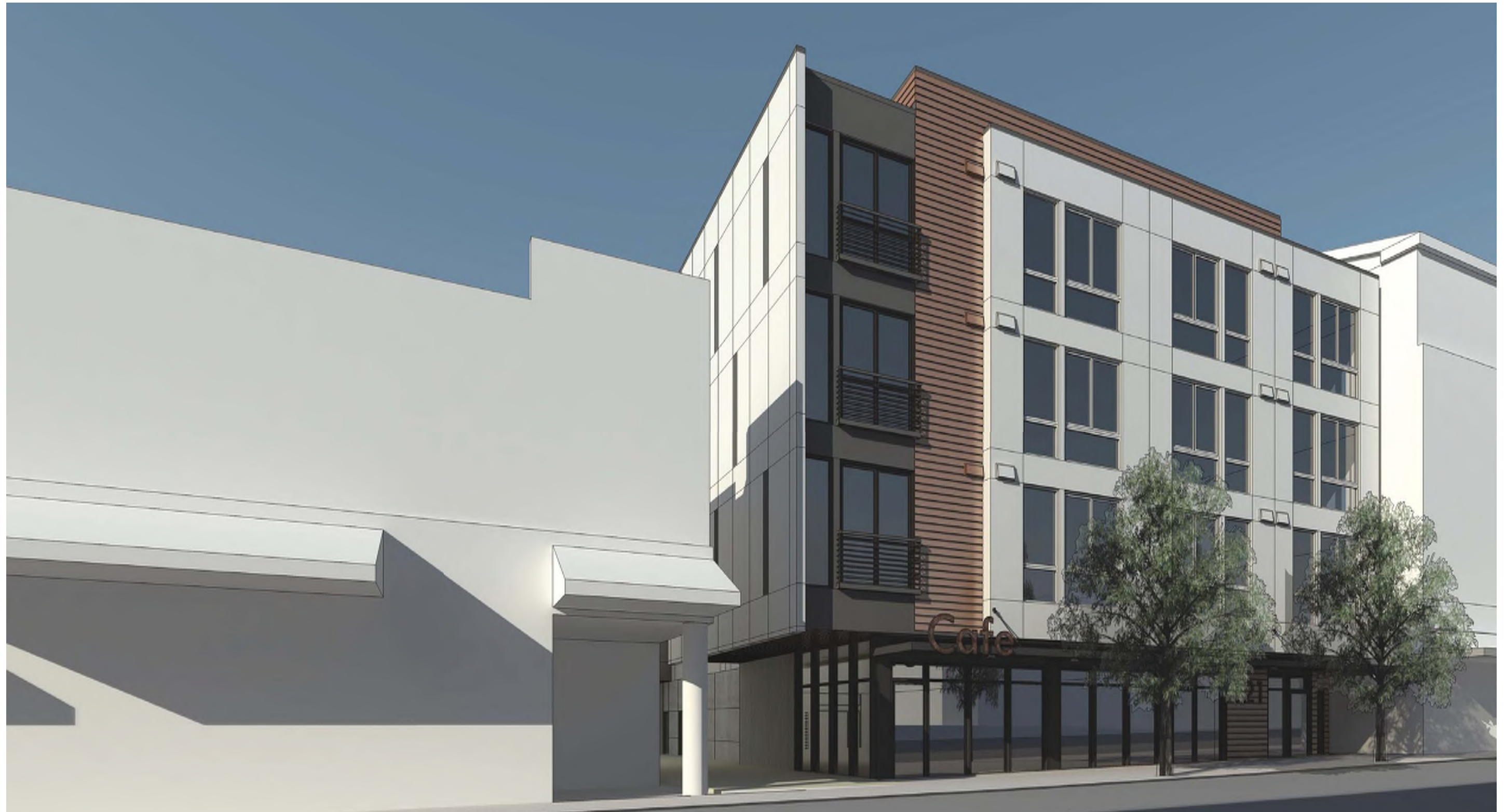
STREET FACADE FROM SOUTH
