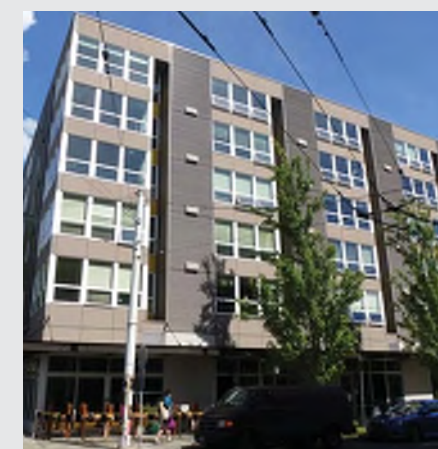
11 APARTMENTS AT E. PINE ST & 15TH AVE CANOPIES & MATERIAL CHANGE DIFFERENTIATE BETWEEN RESIDENTIAL & COMMERCIAL SPACES. WIDE SIDEWALKS PROVIDE COMFORTABLE PEDESTRIAN TRAVEL.
