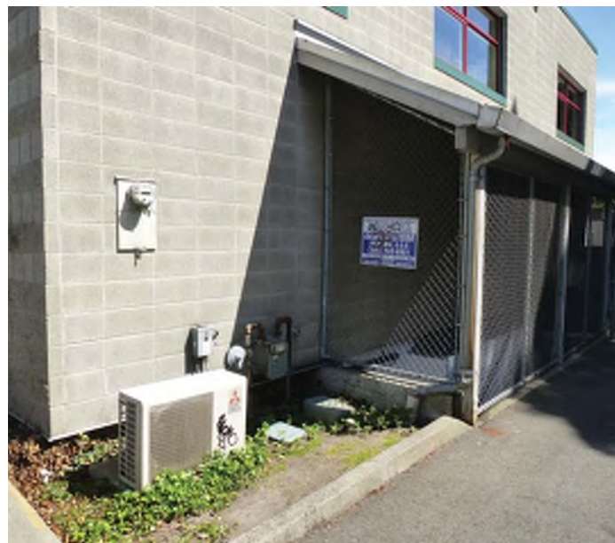
4 BUILDING SOUTH OF SITE
