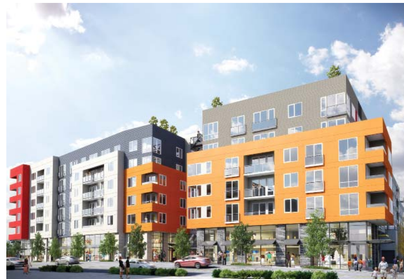
OTHELLO STATION NORTH
