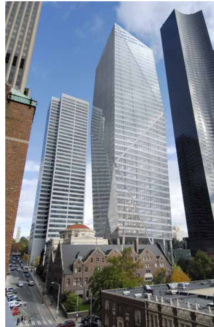
C The Mark (under construction) Completion 2017 | 44 stories | 660'
