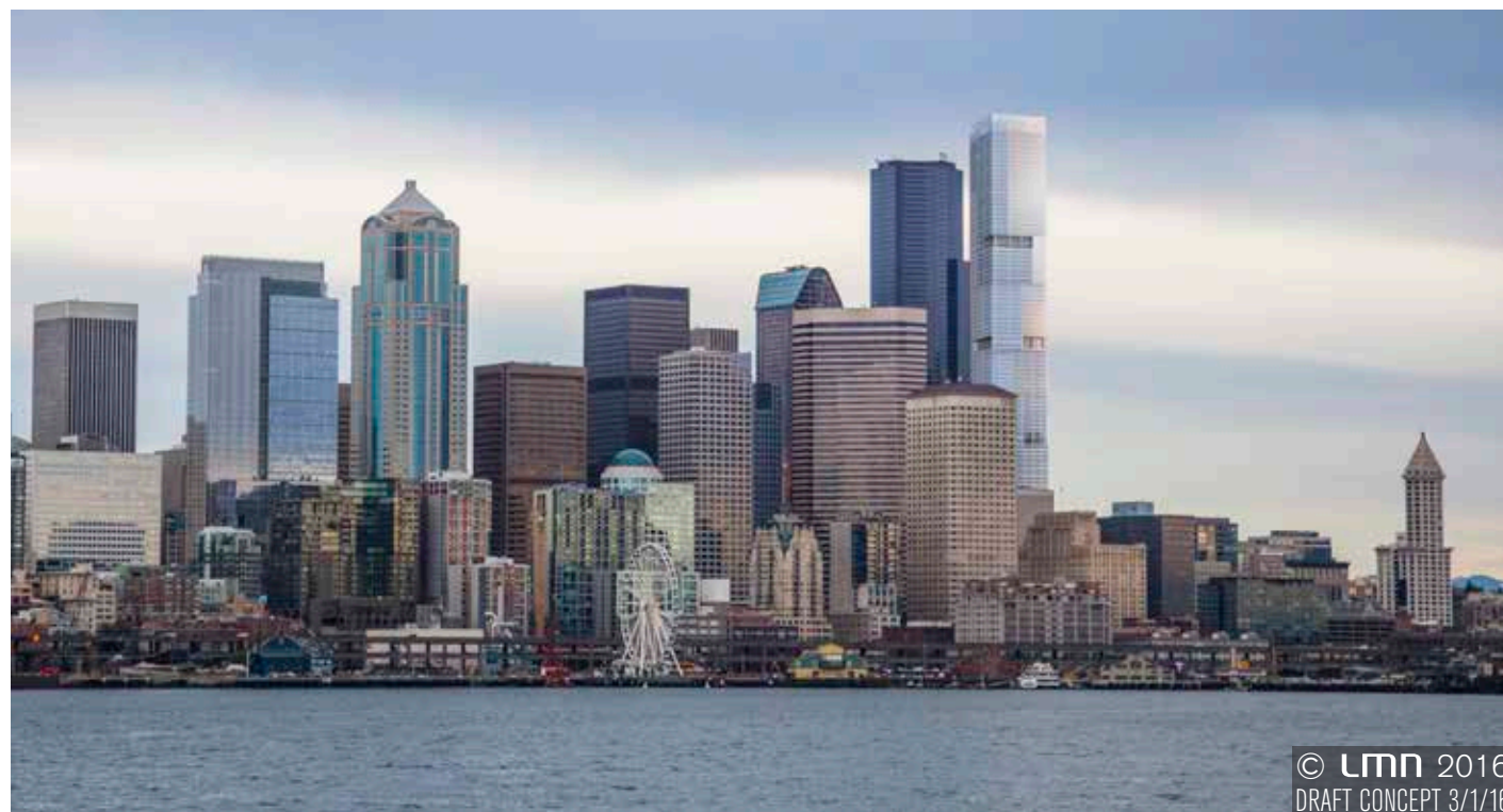
C View from Bainbridge Ferry
