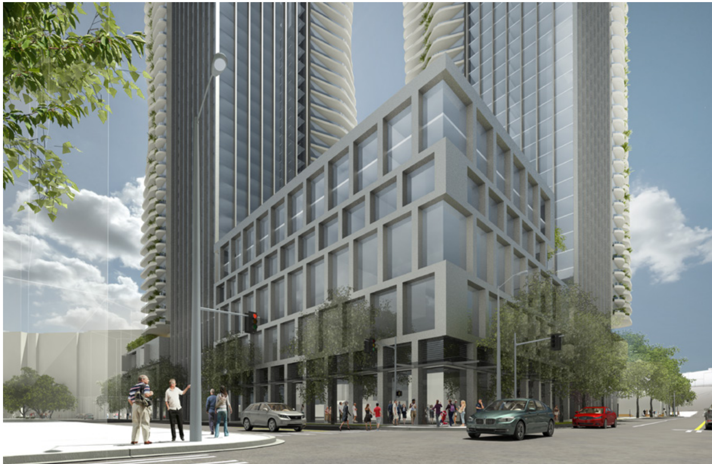
View From Intersection of Stewart Street & Minor Avenue
