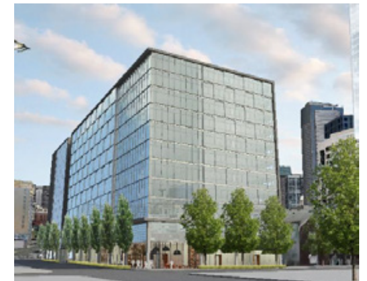
8 1821 Boren Avenue: Under Construction Technology Office and Hotel Building Storeys: 11 (Office), 13 (Hotel)
