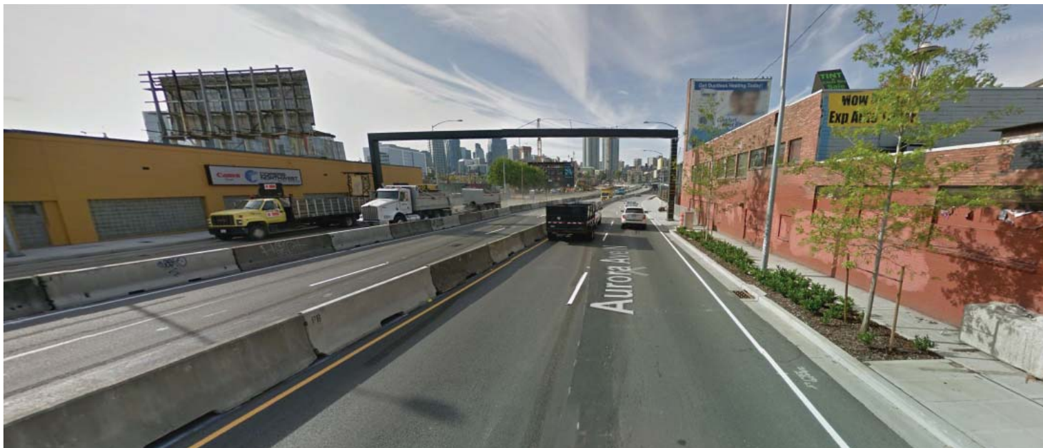
AURORA AVENUE NORTH - LOOKING SOUTH HIGH VISIBILITY OF SITE FROM AURORA AVENUE. HEAVY VEHICULAR TRAFFIC FRONTAGE.
