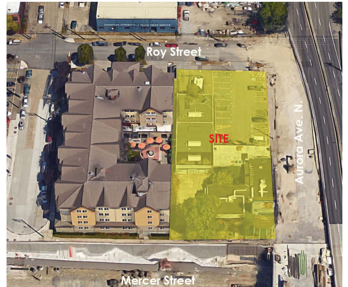
PROJECT SITE LOOKING NORTH ZERO-LOT LINE CONDITION TO ADJACENT HOTEL
