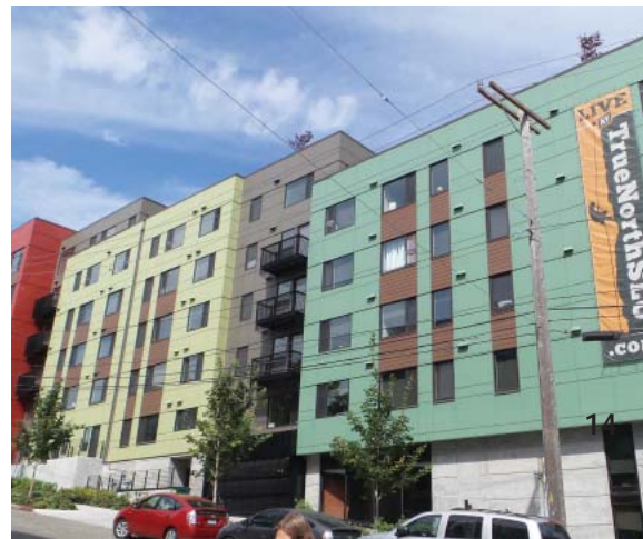
8 TRUE NORTH SLU MIXED-USE APARTMENTS
