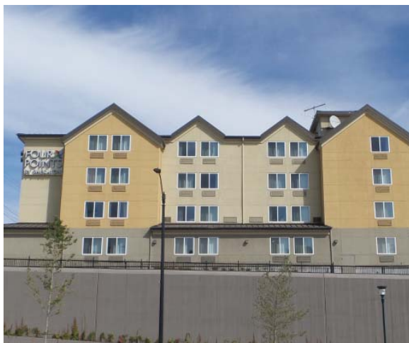
11 FOUR POINTS HOTEL (SAME OWNER AS PROJECT)
