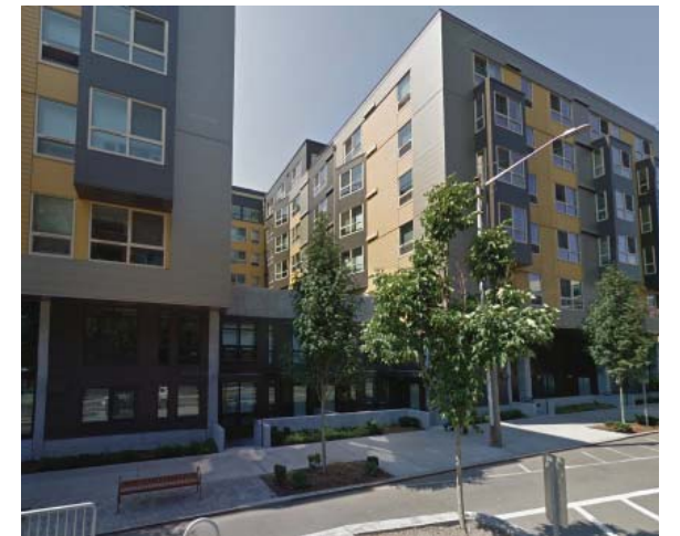
10 UNION SLU MIXED-USE APARTMENTS
