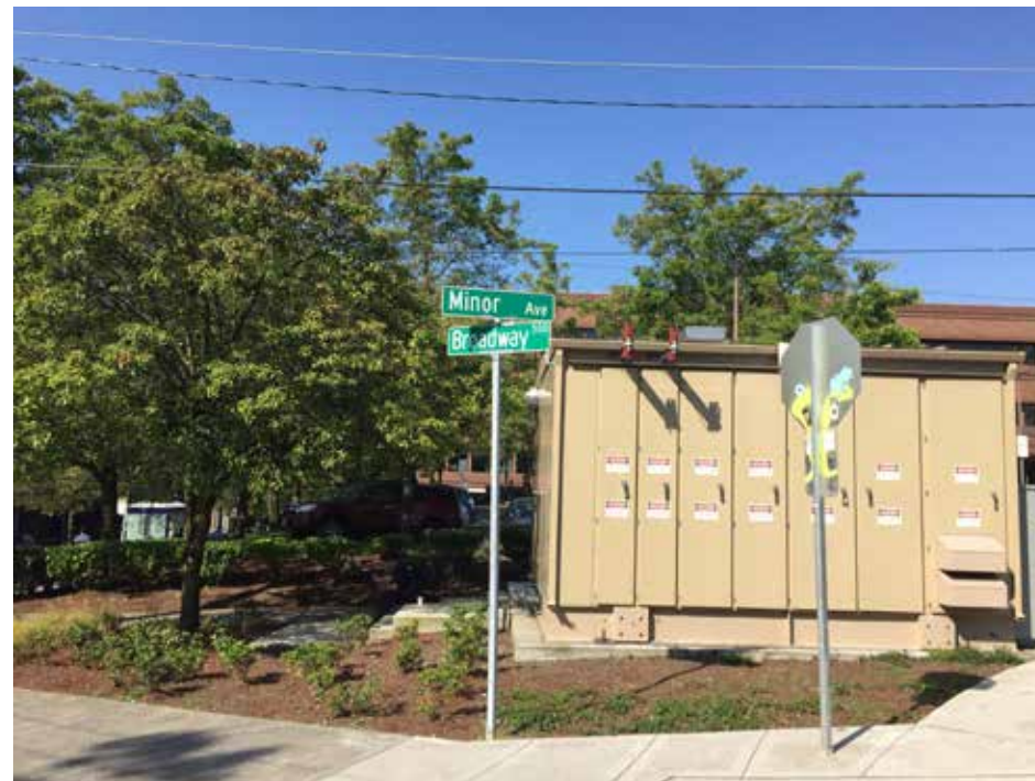
East side of streetcar electrical substation (14' x 17' x 10' H)
