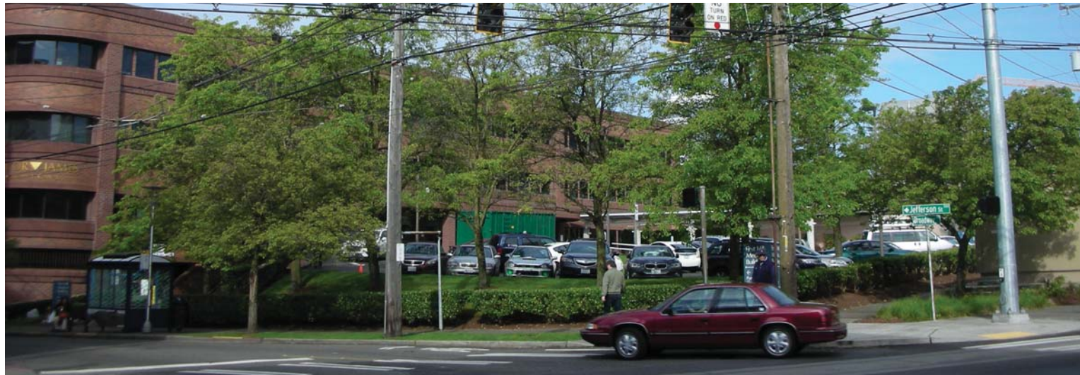
09 SE CORNER OF SITE
