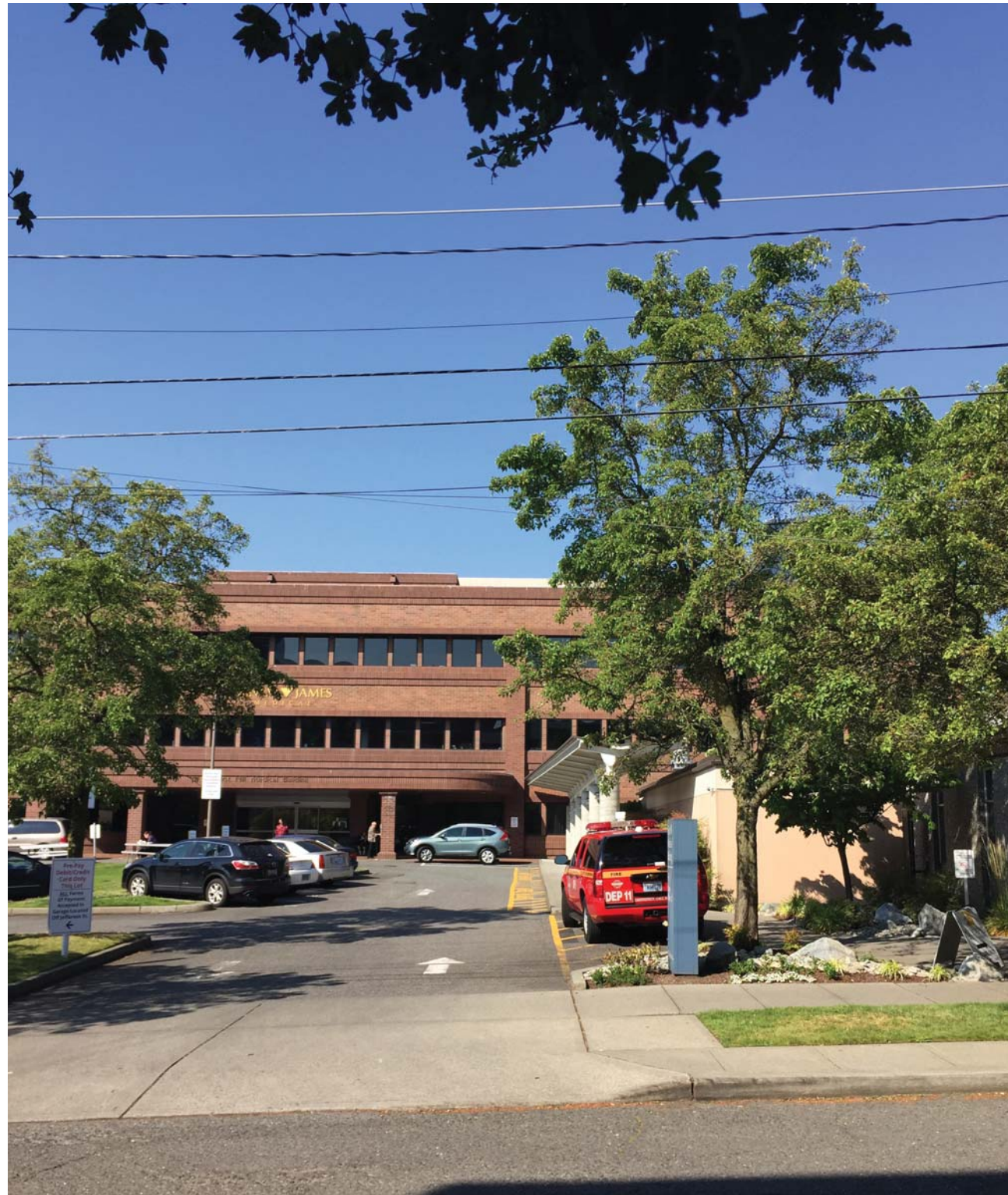
06 EXISTING PARKING ENTRANCE ON MINOR AVE / FRONT DOOR BEYOND
