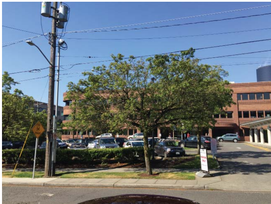
View from Minor showing original and later canopies for drop-off at main entry
