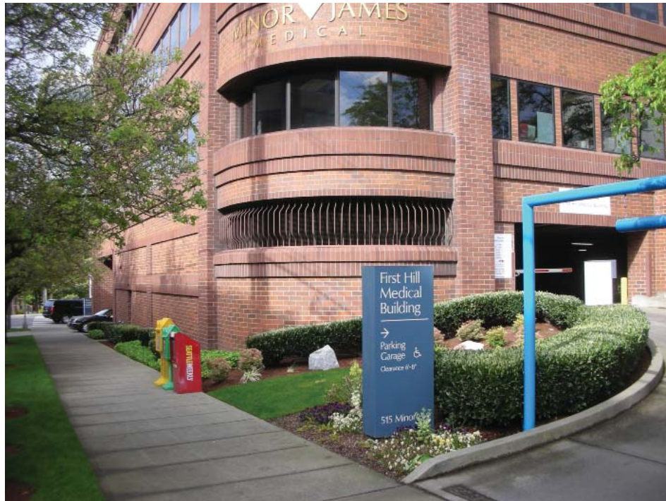
South corner of building showing parking garage entry off Jefferson
