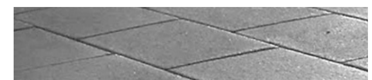
CONCRETE PEDESTAL PAVERS AT COURTYARD
