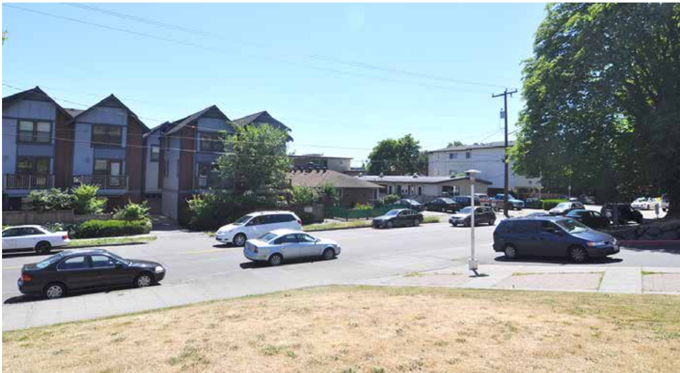
1 View from NE
