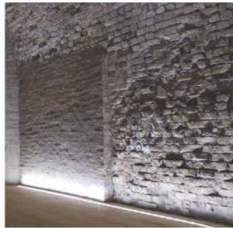
E2 LINEAR LED GRAZER LINEAR LED FIXTURE TO GRAZE WATER FEATURE WALL
