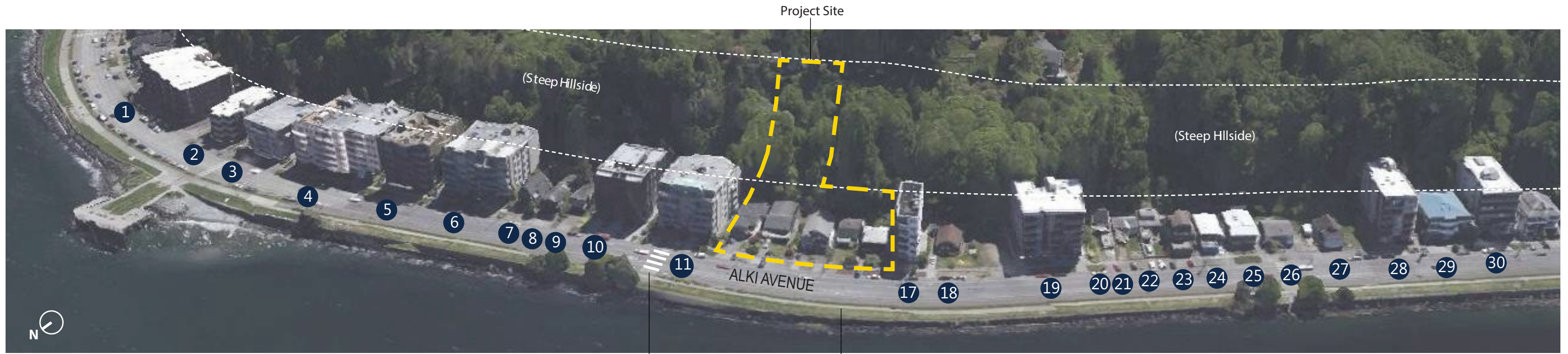
AERIAL VIEW OF ALKI AVENUE SW ALONG NINE BLOCK AREA
