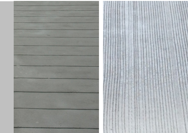
12" band scoring w/ raked finish at vehicular surfaces, medium etch at pedestrian
