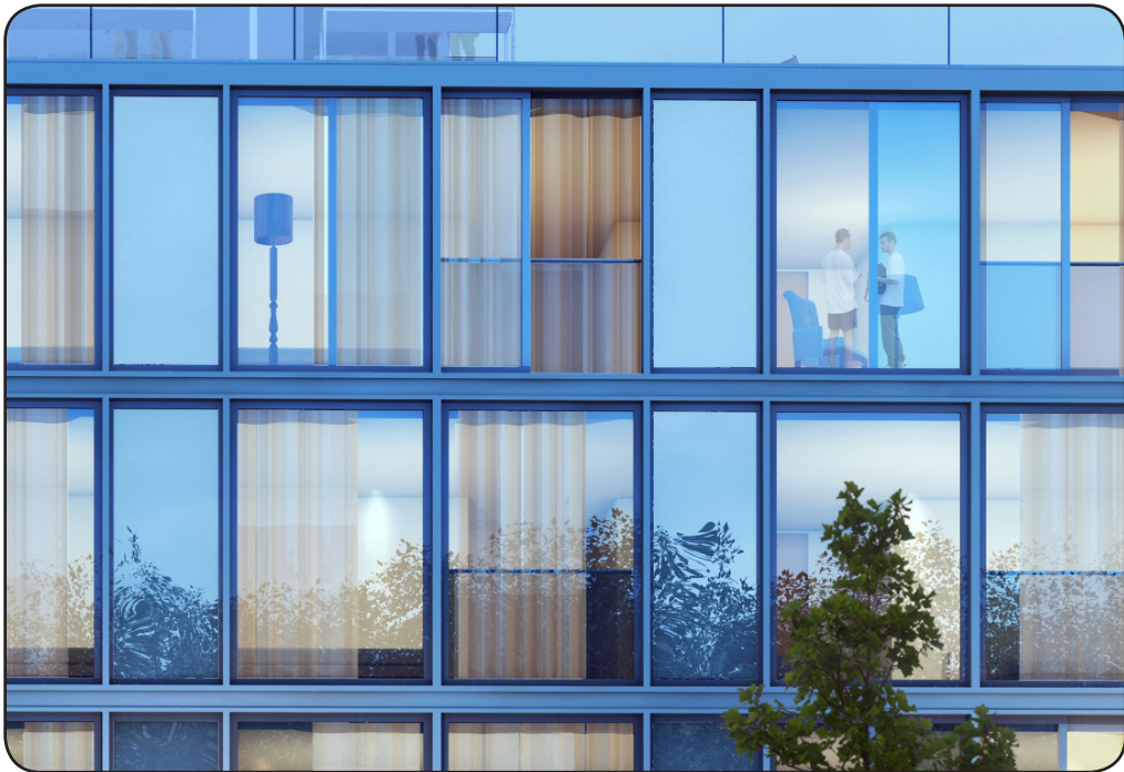
A Material & Screen Translucent glass spandrels will be used to create a continuous glossy facade, allowing the visual language to read as transparent, yet allowing the inhabitants to modulate privacy in their rooms with interior curtain screen.
