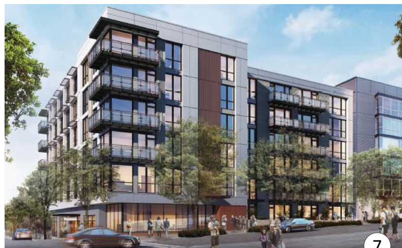
7 Under Construction 124 Denny Way DPD #3015549
