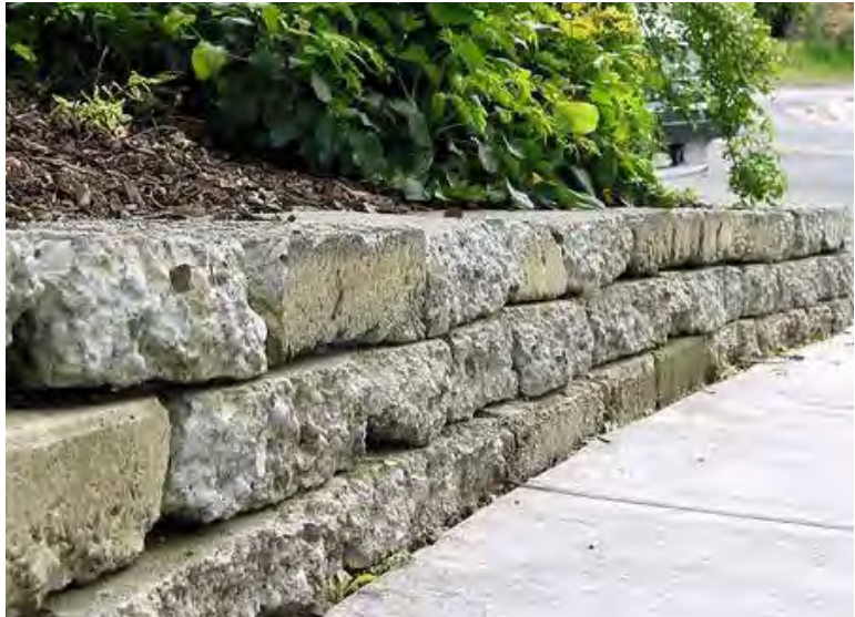
Salvaged concrete rubble wall
