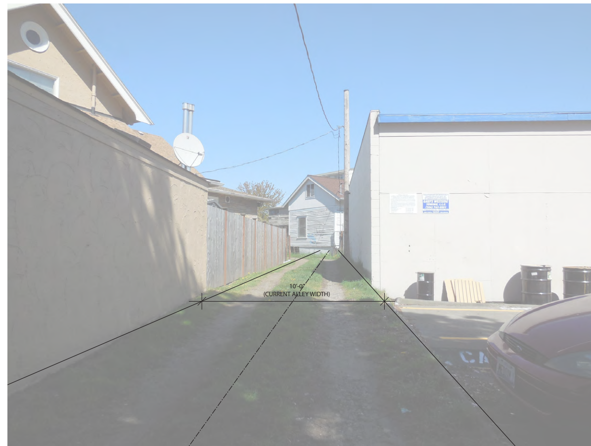
Existing conditions in unimproved alley
