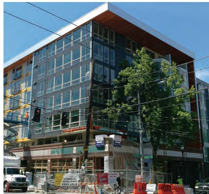
02. 721 E PINE ST | UNDER CONSTRUCTION
