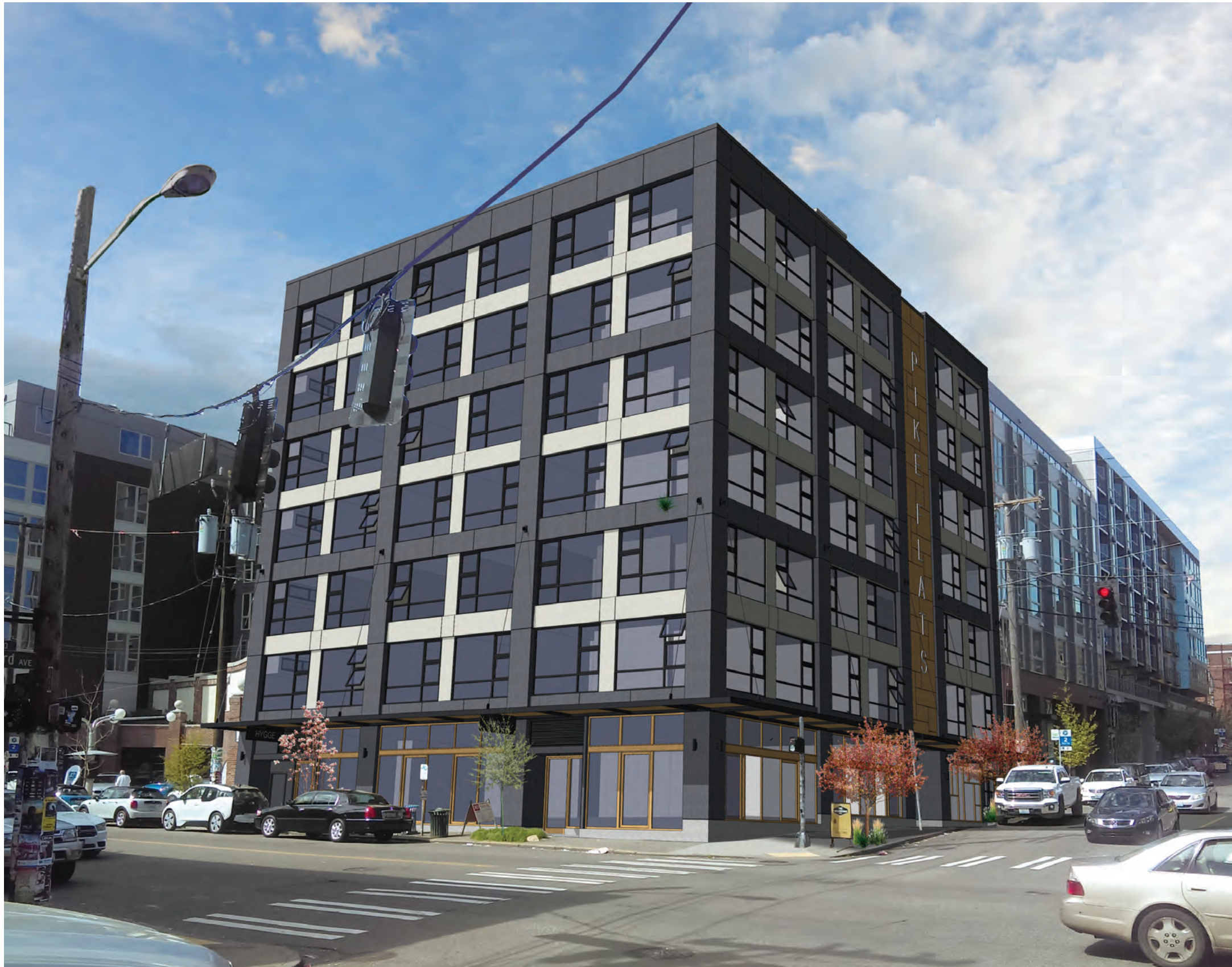
LOOKING NORTHWEST ACROSS INTERSECTION OF PIKE & HARVARD
