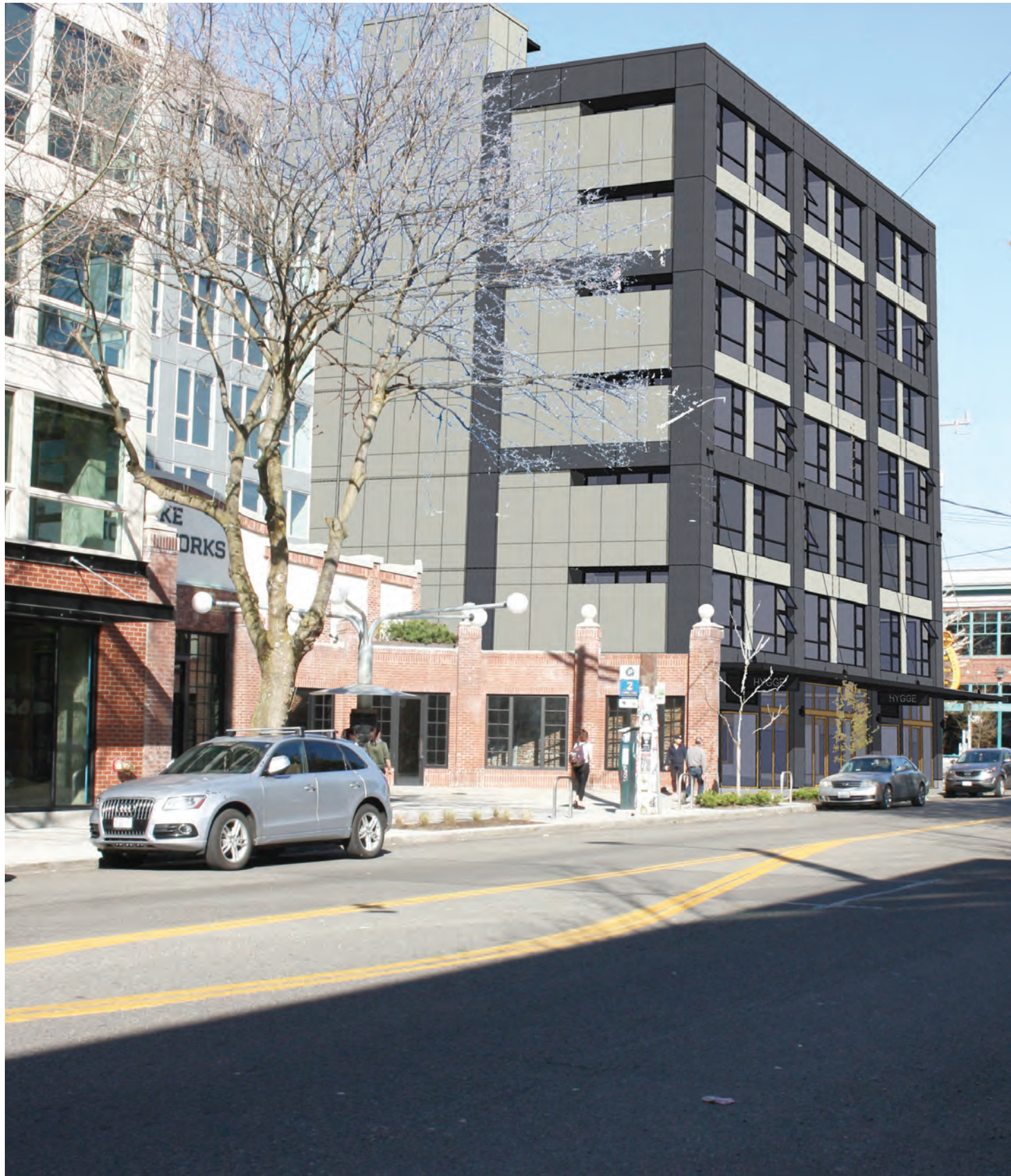
LOOKING NORTHEAST ACROSS PIKE
