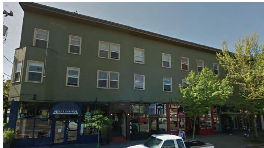
08. BUILDING TO SOUTH OF SITE
