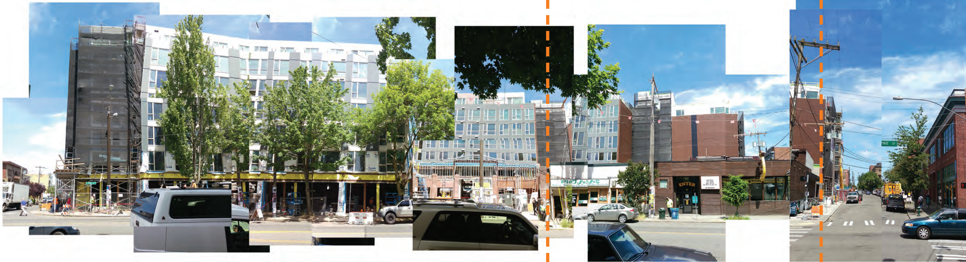
SITE ALONG E PIKE STREET
