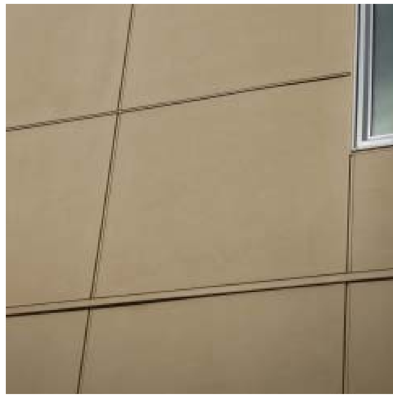
Vertical Reveals & floor flashing
