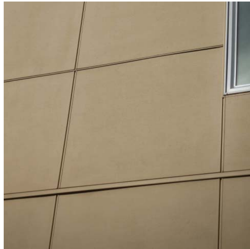
Vertical Reveals & floor flashing
