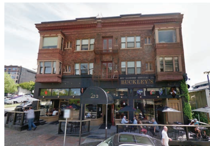
1 Balconies - Traditional Brick Apartment
