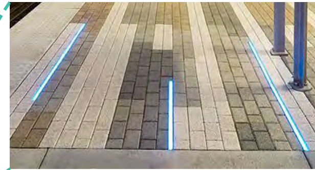
LIGHTING IN SCORED CONCRETE
