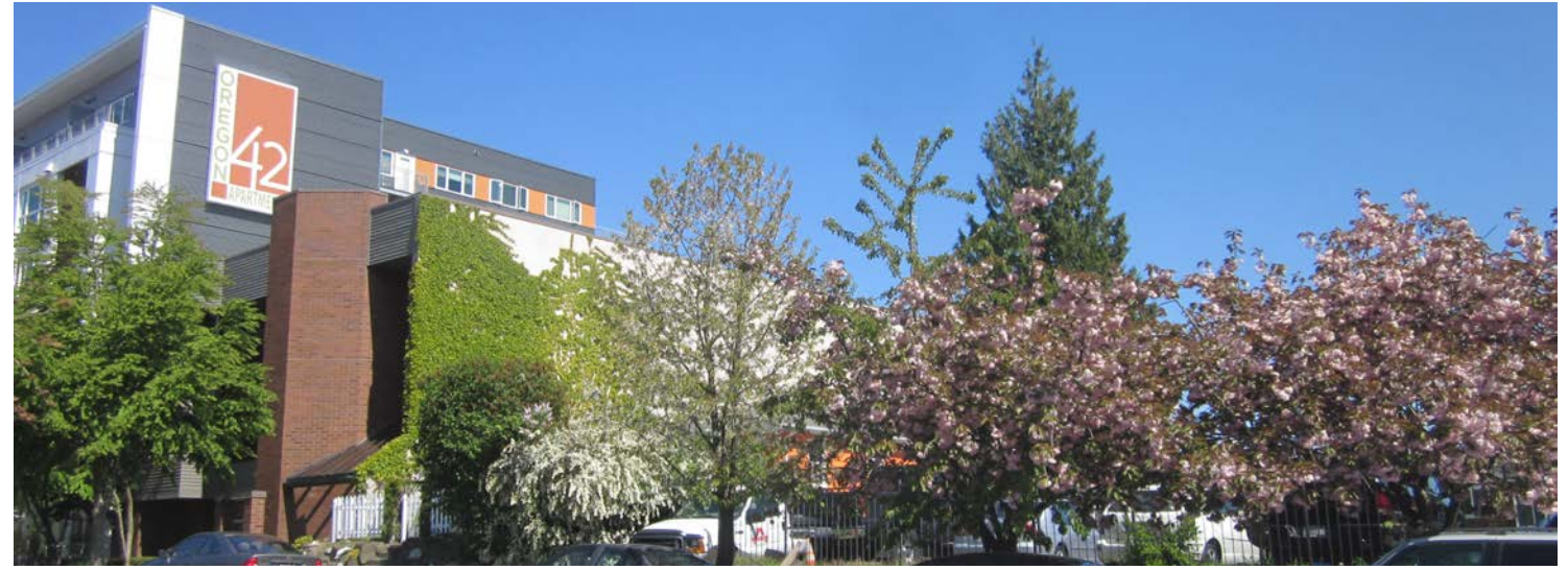
4502 42ND AVENUE SW Oregon 42 Apartments
