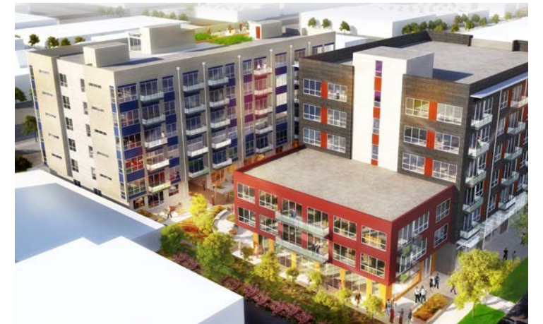
BROADSTONE KOI - LEED-NC CERTIFIED TARGET
