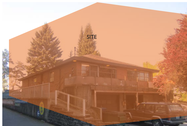
③ PROJECT SITE LOOKING NORTHWEST FROM ALLEY
