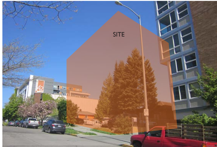
① PROJECT SITE LOOKING NORTH UP 42ND AVE. SW
