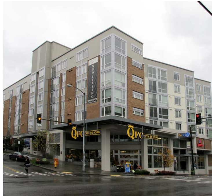
4100 42ND AVENUE SW - CAPCO PLAZA
