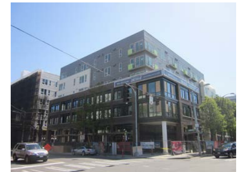
③ JUNCTION 47 (@ CALIF. AVE. SW)
