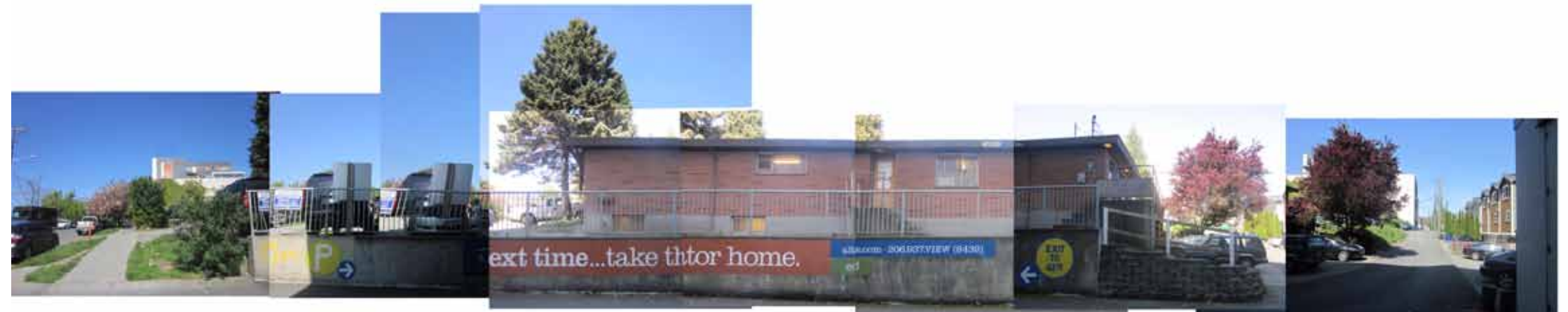
① ALLEY LOOKING NORTH
