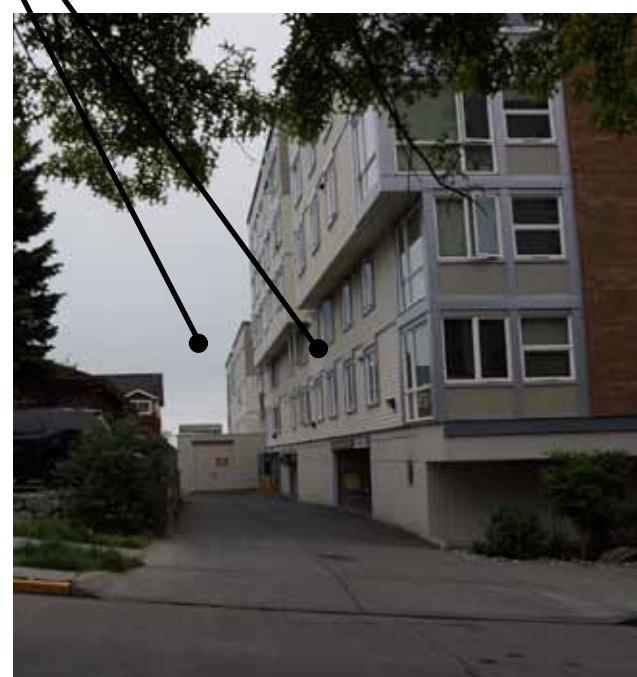
4100 42ND AVENUE SW - SERVICE DRIVE
