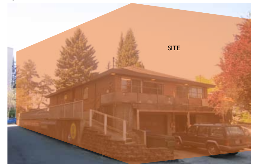
③ PROJECT SITE LOOKING NORTHWEST FROM ALLEY
