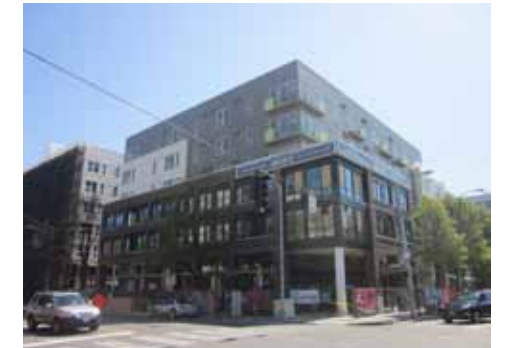
③ JUNCTION 47 (@ CALIF.AVE SW)
