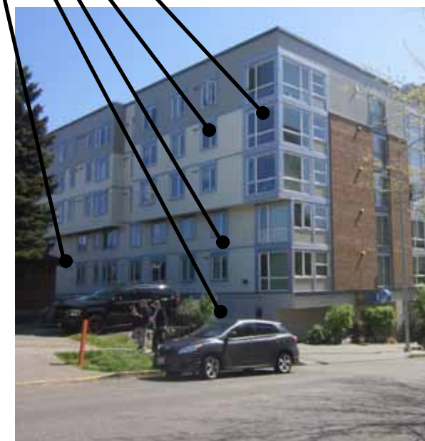
4100 42ND AVENUE SW - NW CORNER
