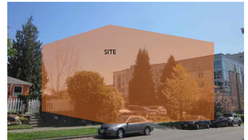
② PROJECT SITE LOOKING SOUTHEAST DOWN 42ND AVE SW
