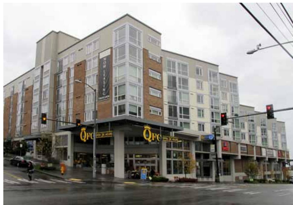
4100 42ND AVENUE SW - CAPCO PLAZA
