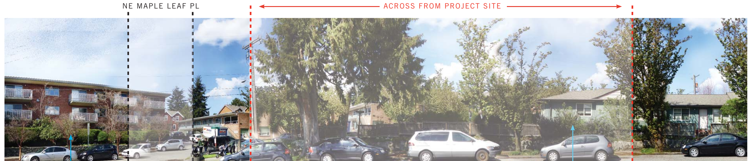
CONDOS 3-Story Building
