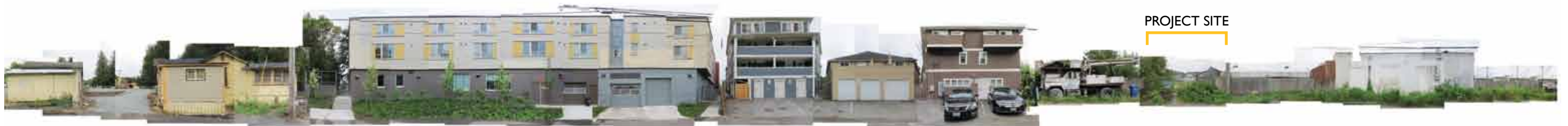
③ ALLEY LOOKING WEST TOWARDS PROJECT SITE
