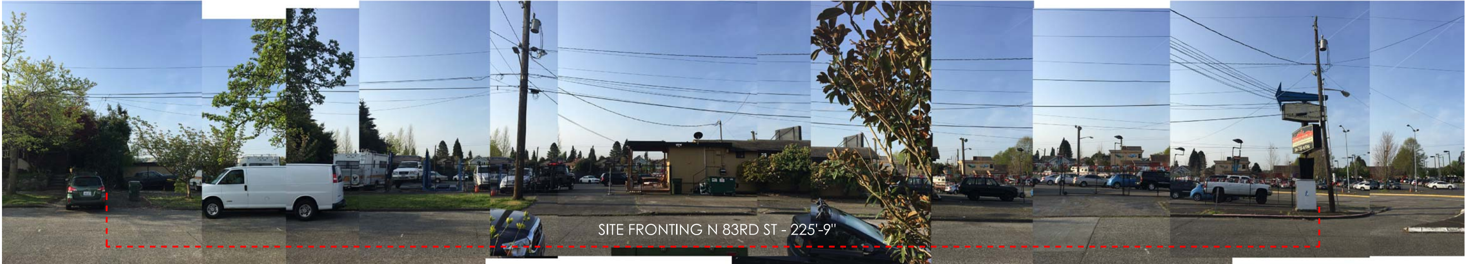
N 83RD ST MONTAGE - VIEW SOUTH TOWARDS SITE
