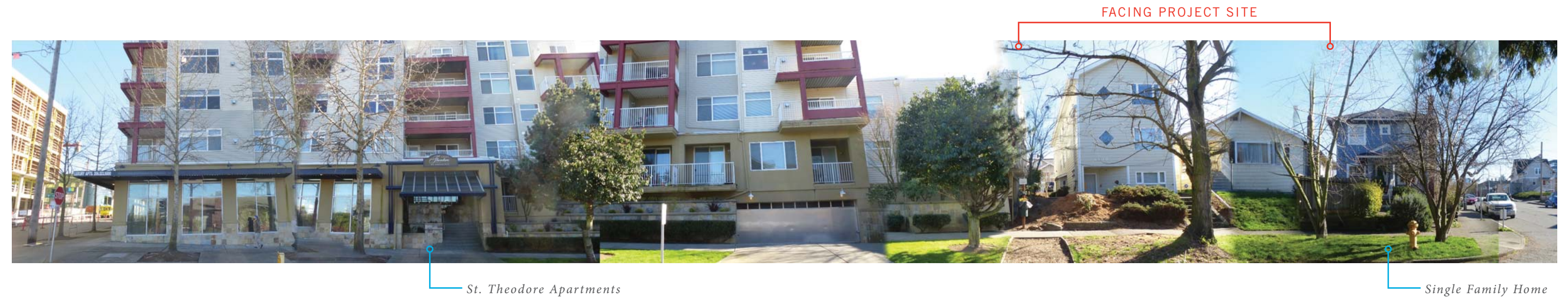
A. 9TH AVE NE, LOOKING EAST
