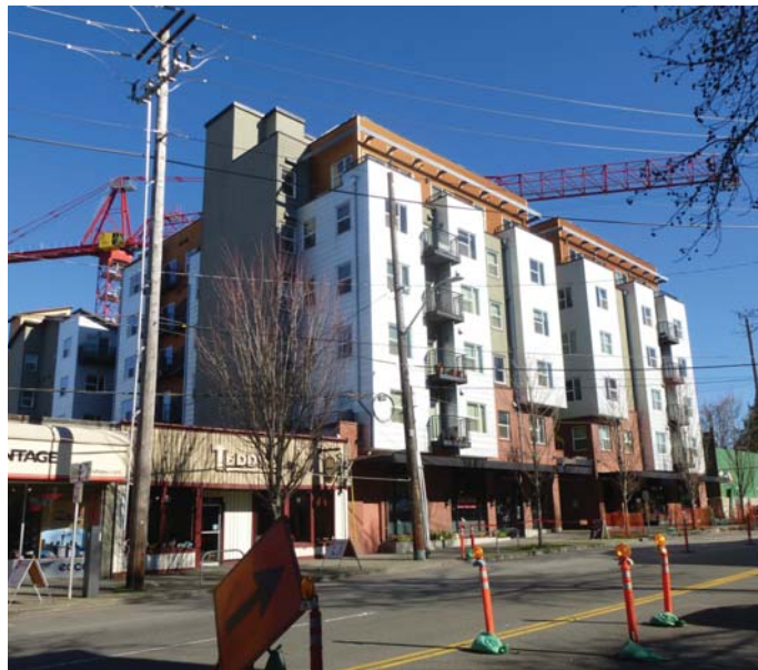
5 APARTMENT COMPLEX AT NE 65 TH ST, NE OF SITE
