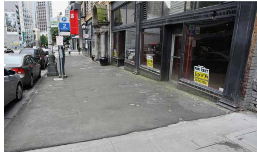
Sidewalk is mix of materials and textures including concrete, asphalt, moss and pigeon droppings.
