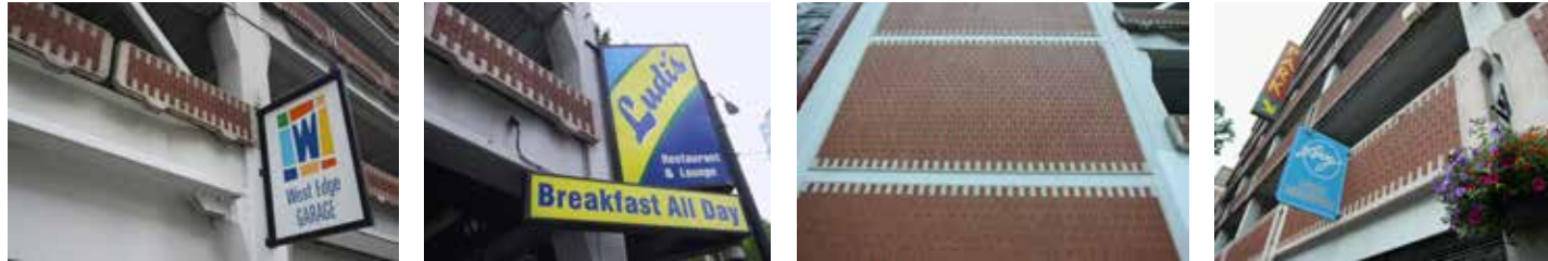
Protruding signage and unusually oriented masonry adorns both west & south facades.
