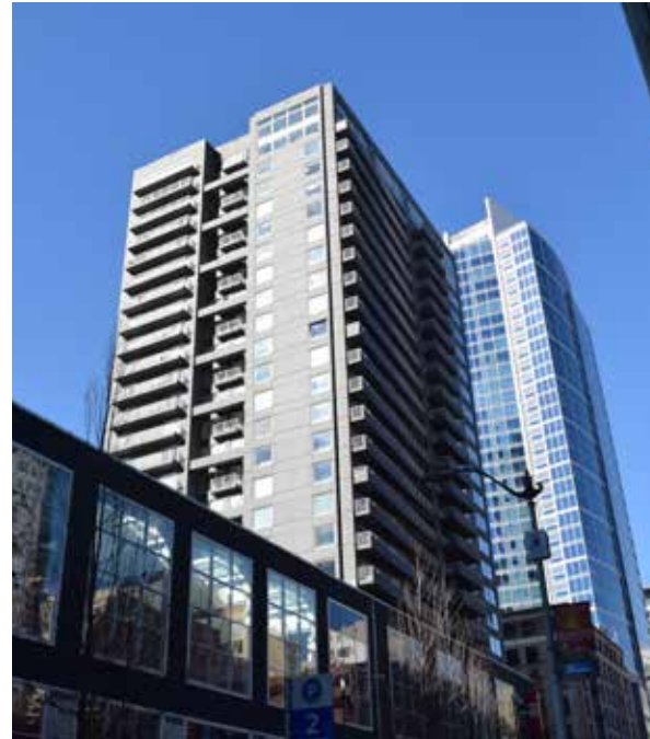
1991 / 260' / 25 Floors / 190 Units / Residential
