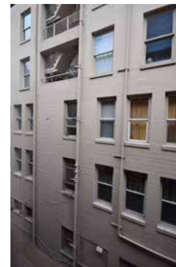
Lower west (alley side) facade of Fischer Studio Building
