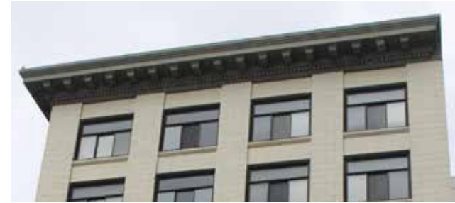
Top of Haight Building
