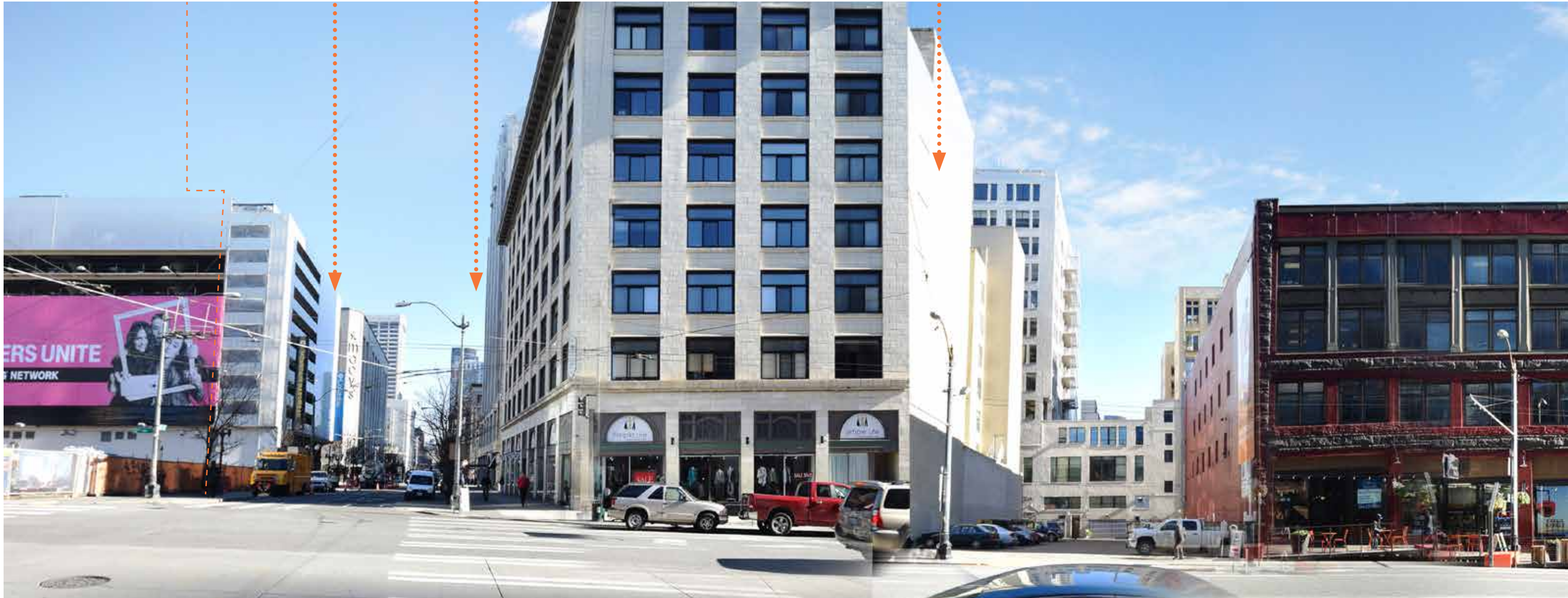
16 2nd + Pine Future Tower Site (Under Construction) #3014773 — see page 11
