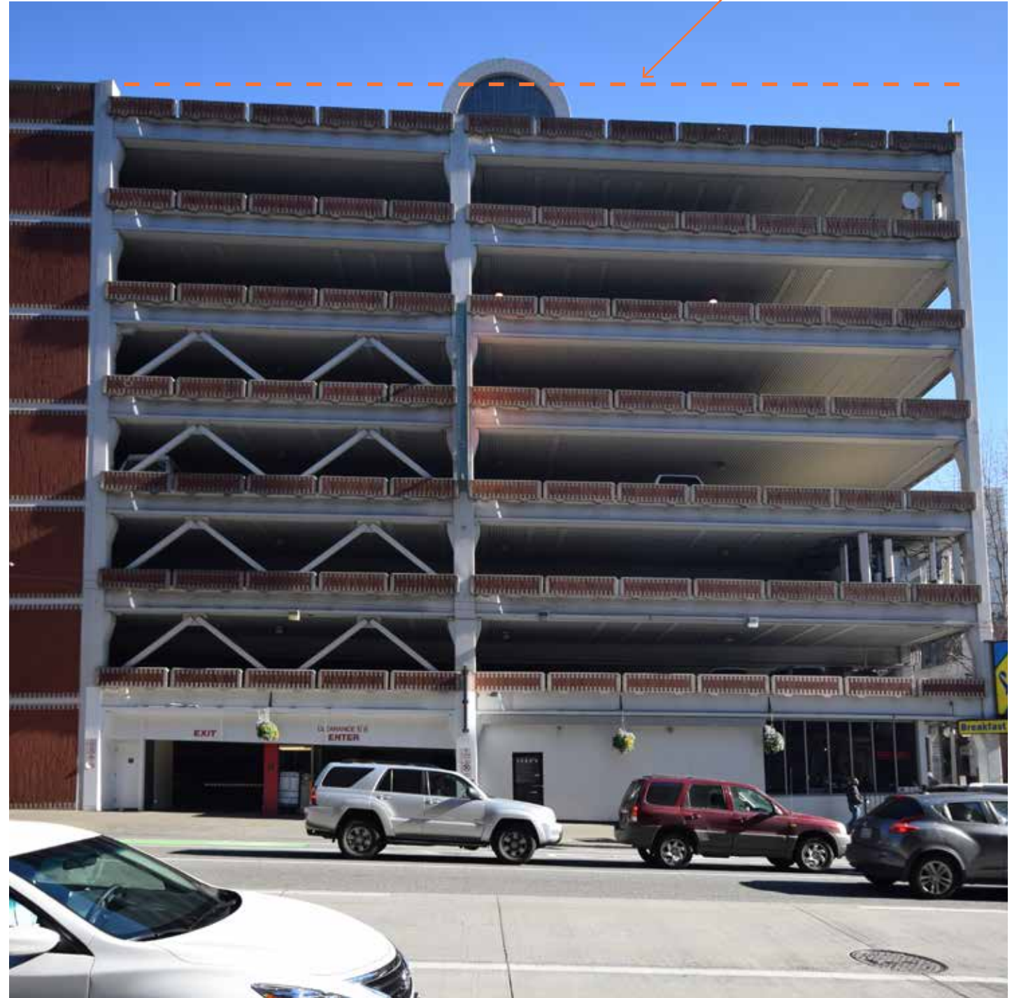
Limited street-level transparency at the garage. The curb cut, with in-and-out traffic interrupts pedestrian flow along 2nd. The architecture of the garage presents limited design cues to work with. Note that the floor plates are sloped.
