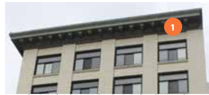
Top of Haight Building
