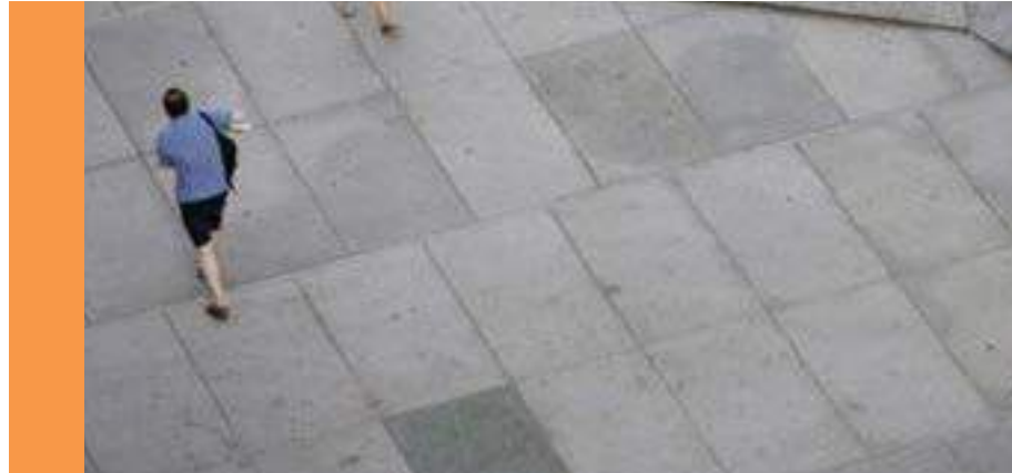
Sandblasted CIP Concrete Paving
