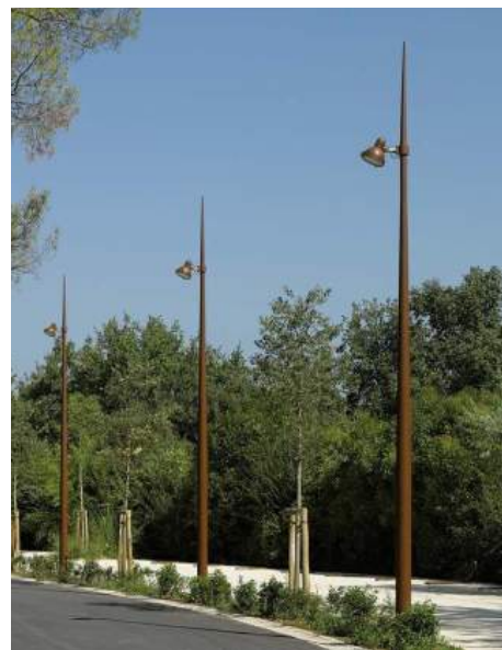
Indirect plaza lighting
