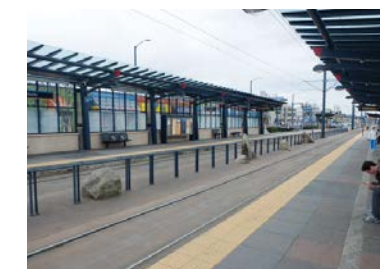
Othello Light Rail Station
