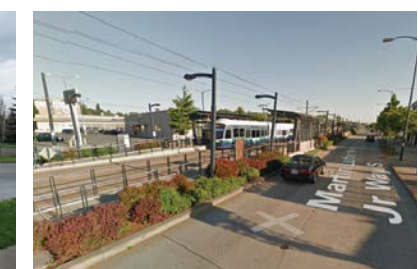
Othello Light Rail Station
