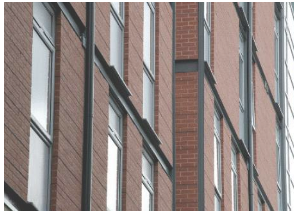
BRICK WITH STEEL LINTELS
