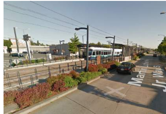
02 Othello Light Rail Station
