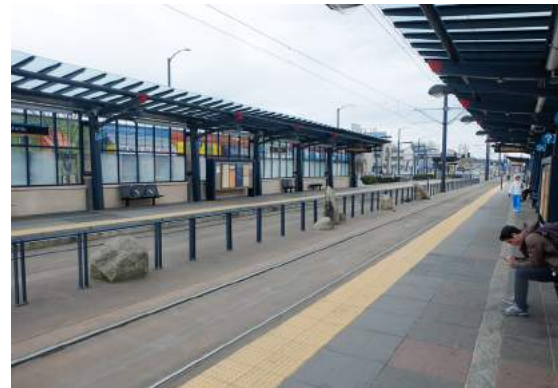
03 Othello Light Rail Station
