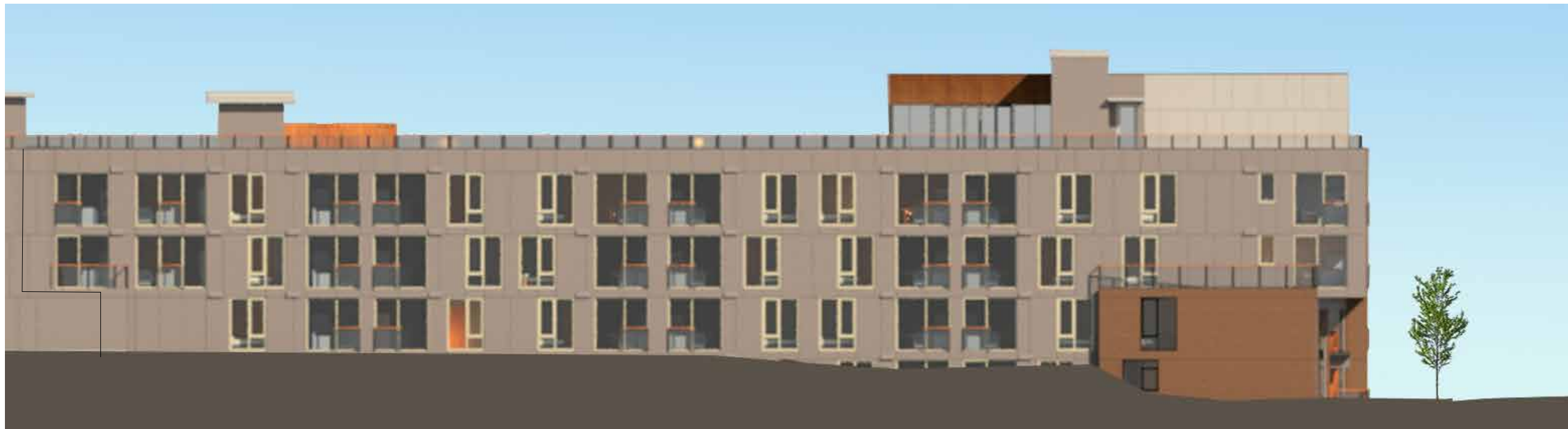
East (38th Ave S) end
