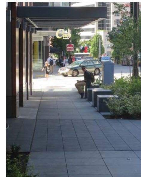
1 Sandblast, Sawcut Joints
