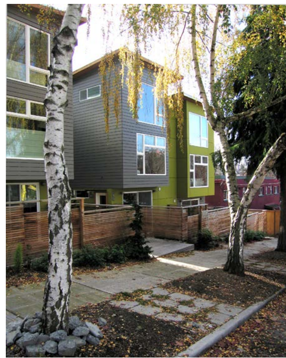
⑤ 1411 E. Fir St. (View from street)
