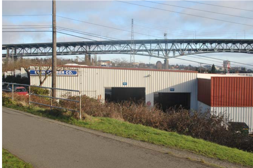
Bridge and Burke Gilman Trail
