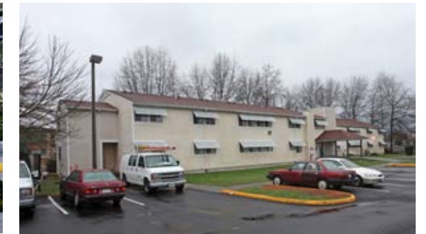
6- HOLLY COURT 3824 S MYRTLE ST | APARTMENTS Holly Court is a low income housing complex by the Seattle Housing Authority. Project site and apartment complex are divided by a tree barrier.
