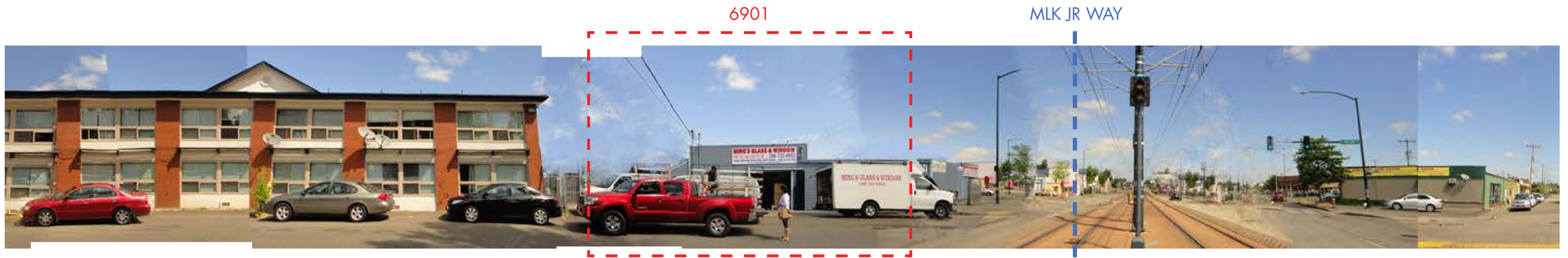
C- VIEW ALONG S. WILLOW STREET FACING NORTH
