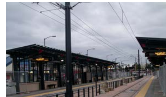
8- OTHELLO STATION 7100 MARTIN LUTHER KING JR WAY S | STATION Frequently used lightrail station that connects Othello to downtown Seattle. Located inbetween the street.
