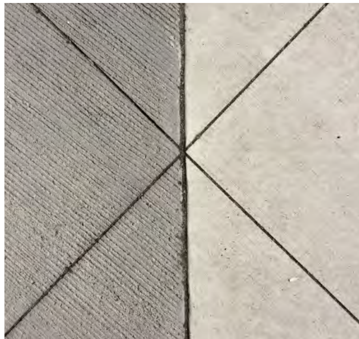
Bell Street Paving
