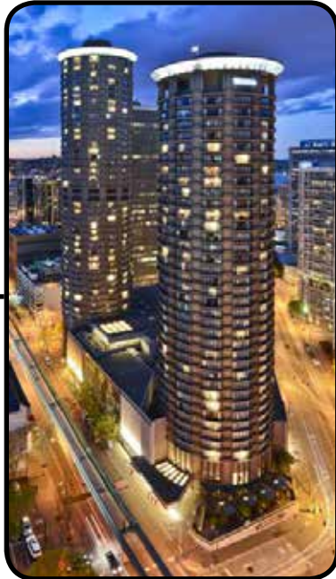
Westin Towers Seattle John Graham & Co. - 1969-1982 40 & 47 Floors
