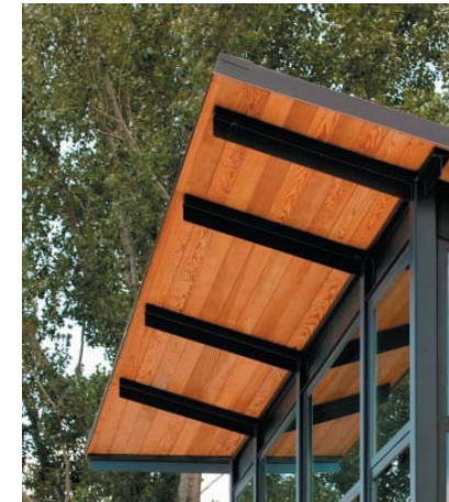
RETAIL AWNING: EXPOSED STEEL FRAME AND STAINED WOOD T&G SOFFIT
