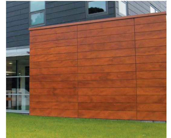
WOOD SIDING: HORIZONTAL PANEL CONFIGURATION WITH EXPRESSED HORIZONTAL REVEALS. ALIGNMENT WITH WINDOW "PUNCHED" OPENINGS
