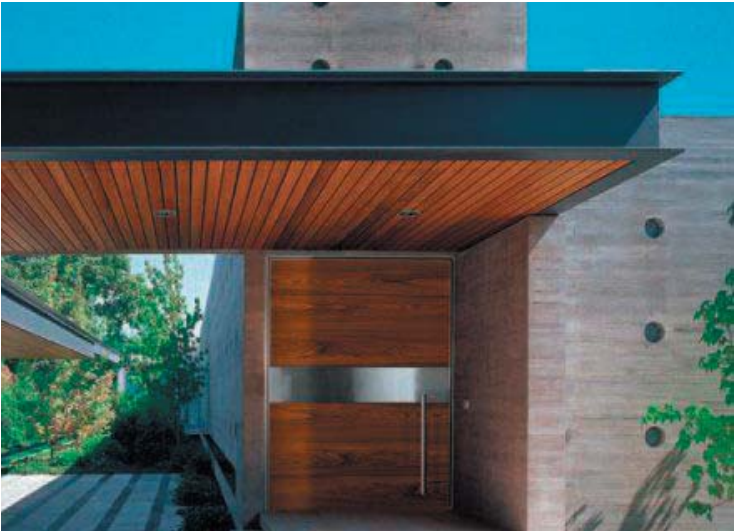
ENTRY AWNINGS: EXPRESSED STEEL C-CHANNEL FRAME WITH FLUSH SOFFIT AND RECESSED LIGHTING
