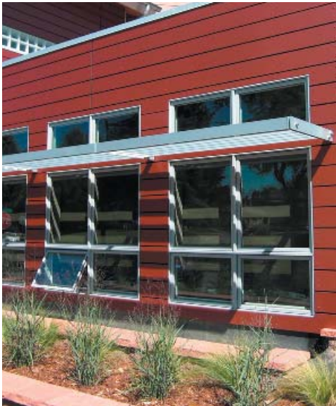
LIVE/WORK AWNINGS: STEEL SCREENING ALLOWING FILTERED LIGHT ALONG COMMERCIAL USE
