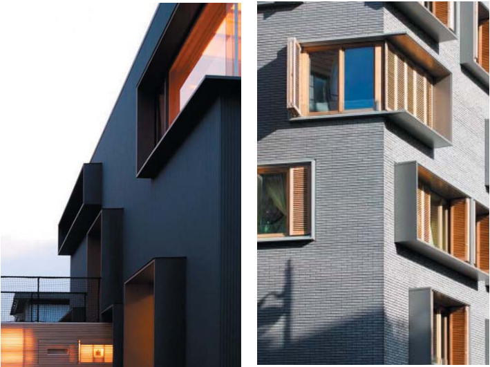
FENESTRATION SURROUND: DEEP STOREFRONT FRAMES AT FEATURE LOCATIONS TO EXAGGERATE PUNCH OPENINGS
