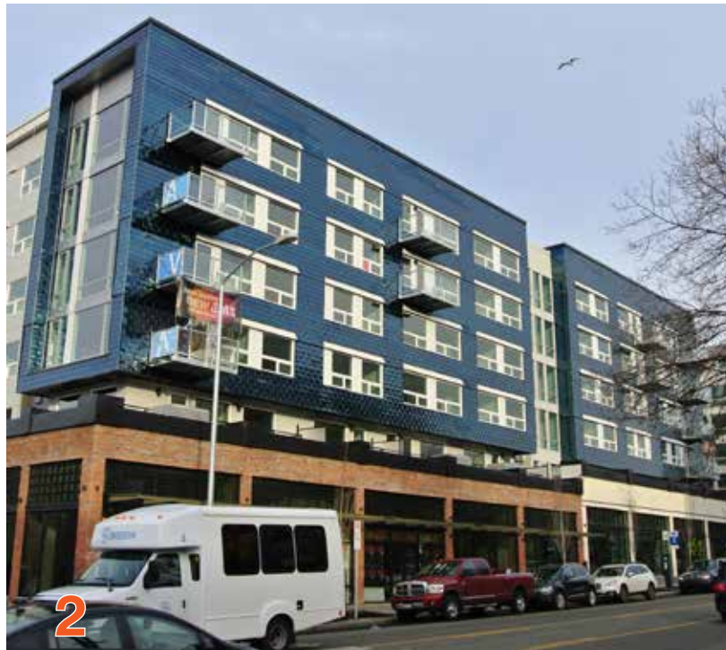
2 AVA CAPITOL HILL (UNDER CONSTRUCTION)
