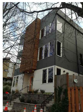
F Modern design w/ use of white Hardie Panel sheets, gray horizontal Hardi Plank, & horizontal wood siding
