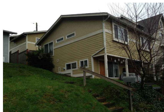
Facing northwest from Fauntleroy Way SW toward duplex at 5911
