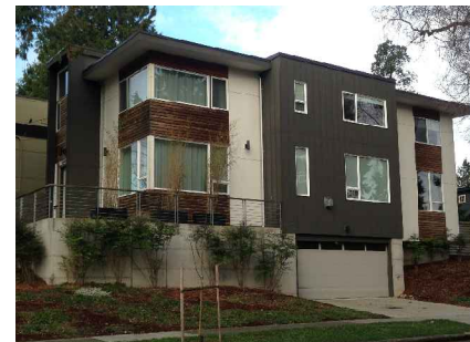
C Modern design w/ use of gray & white Hardie Panel sheets, & wood horizontal siding
