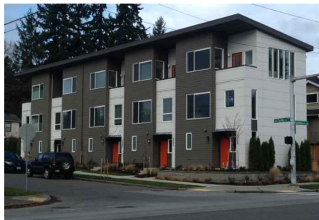
B Modern design w/ use of Hardie Panel sheets, horizontal Hardi Plank, shed roof & deck on 3rd flr
