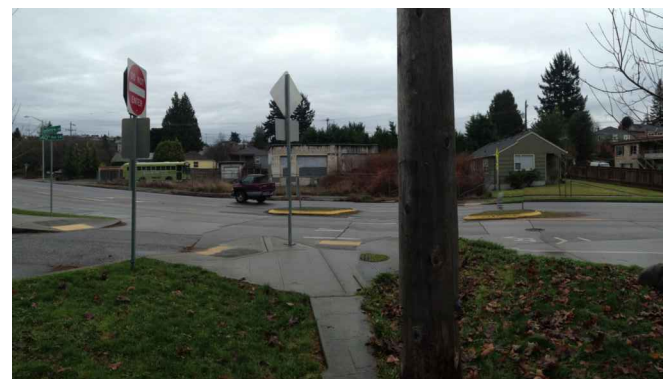
Crosswalk view facing east toward Fauntleroy Way SW
