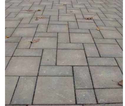
permeable paving in front of rear units
