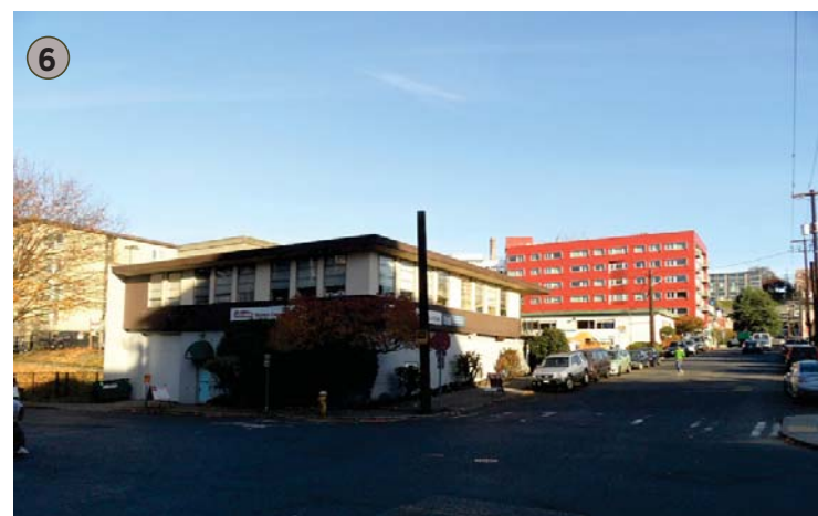
SOUTHWEST VIEW OF SITE A
