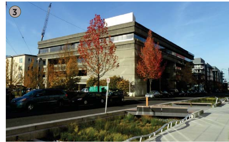
VIEW OF THE PONTIUS BUILDING
