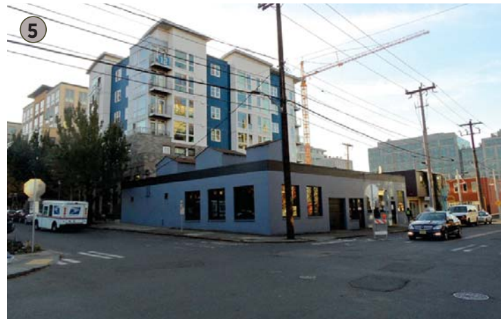
VIEW OF ALCYONE APARTMENTS
