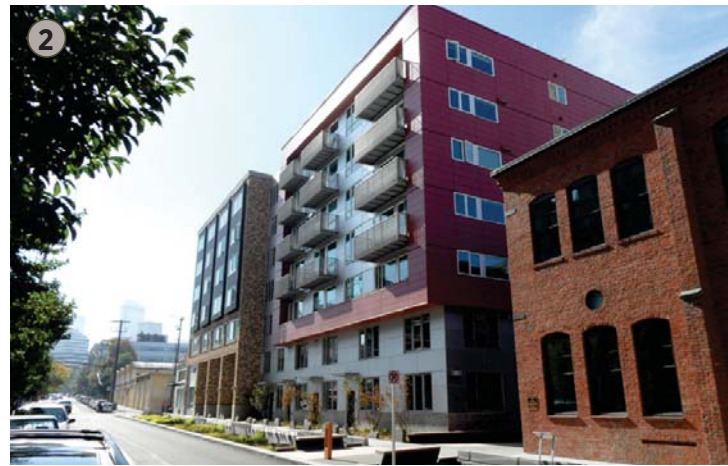
VIEW OF STACK HOUSE
